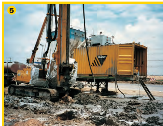
4) MCM 2500 mixing plant with pump container. Mariaposching/Deggendorf, Germany.
