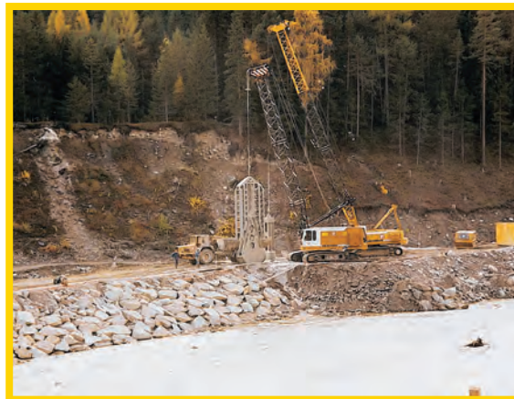
3) MCM 5500 mixing plant for diaphragm wall construction. Hamburg, Germany.
